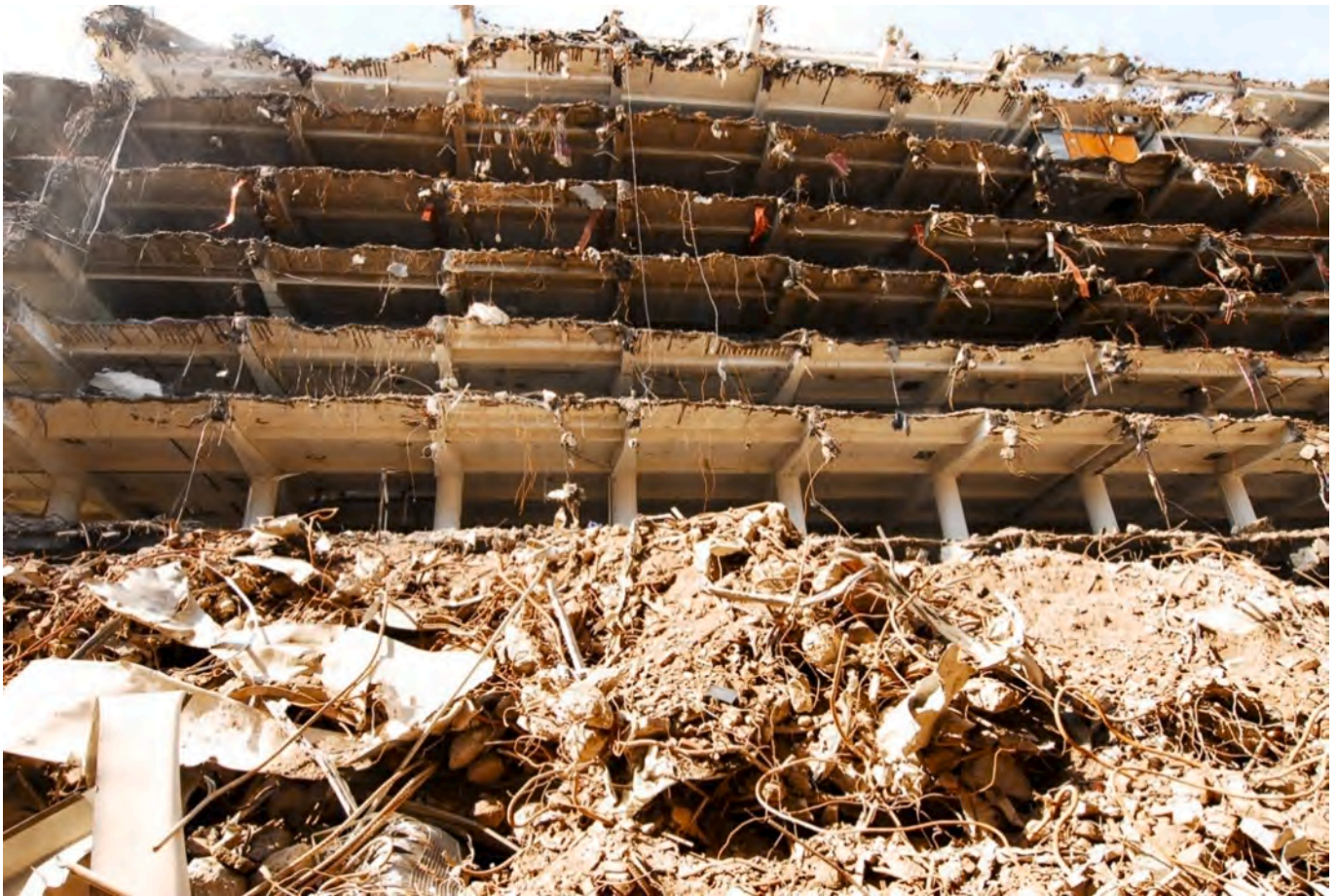
Fig. 3. Demolition in Brussels. Source: author's personal archive.
