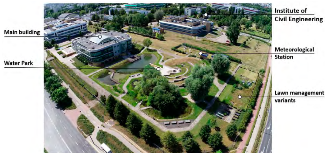
Figure 2. View of the Water Center of SGGW with the water park.
