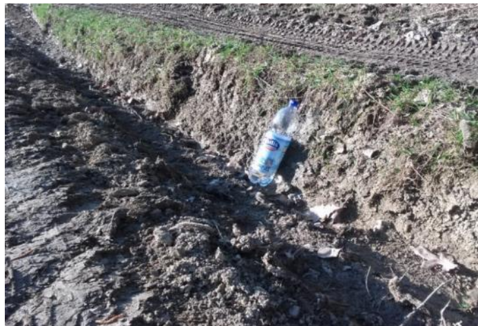
Figure 7 Influence of water erosion on unpaved field road
