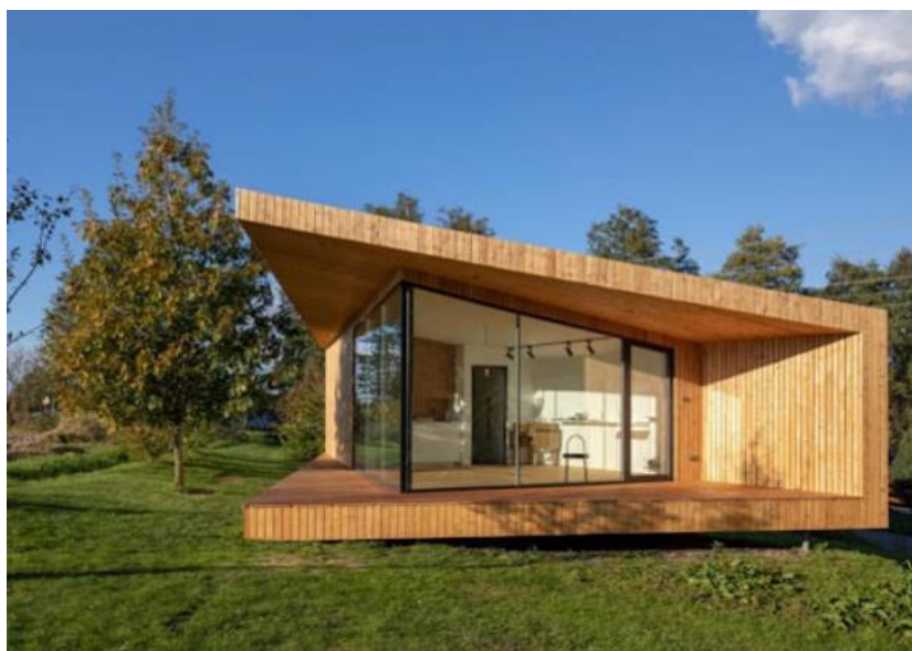
Fig. 5: Example of a timber building based on earth screws (Chytré základy)
